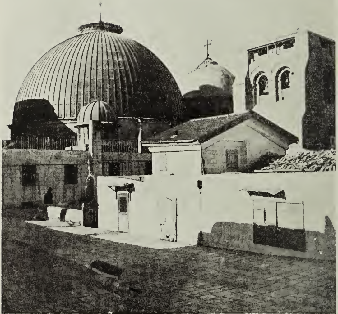
On the roof of the Church of the Holy Sepulchre is a street wider than many in the city below
